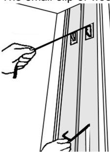
Pass a piece of string with a small weight at the end over the first pulley and allow it to drop to the bottom of the jamb. Attach the other end of the string to a
